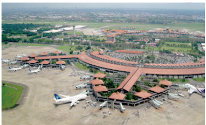
Indonesia Airport Control System
